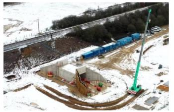
The work is part of the first phase of the A4095 road realignment project, which will see two structures built to enable access both over (a new bridge) and under the railway (pedestrian underpass), connecting two sides of a new area of housing in north-west Bicester.
